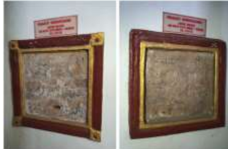
Figure 10 The inscription containing Candrasengkalan is now eroded (Doc. Da'iul Umam Karim: 2021)
