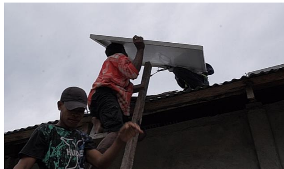
Figure 5. Installation of the Cortagrid system with the Tiflean village community
