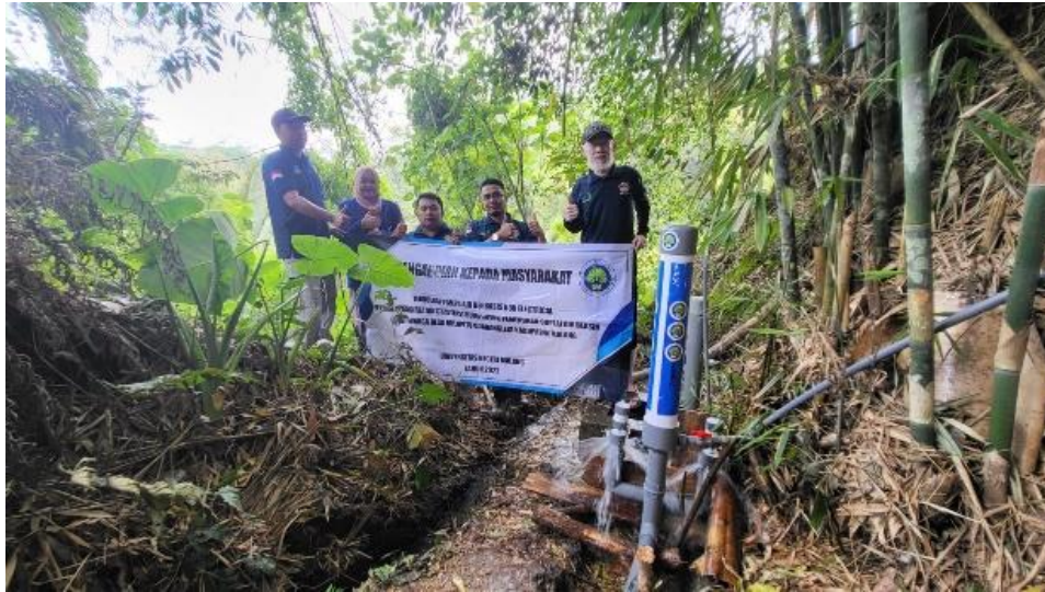
Figure 3. Implementation of Water Pump
