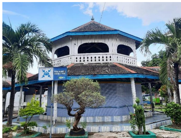
Figure 4: The roof of the ablution place at Sultan Muh. Salahudin mosque is octagonal.
