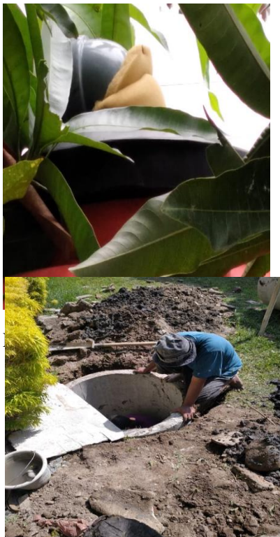
Figure 5. Infiltration Wells
