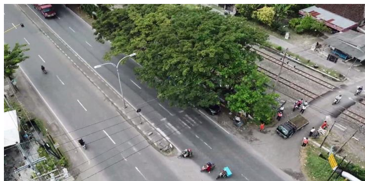
Figure 3. JPL 295 is not equipped with barrier gates
